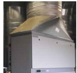
Example of duct installation
